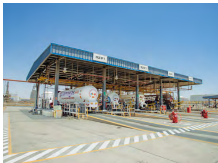
Land cargo terminal, Pisco, Peru
